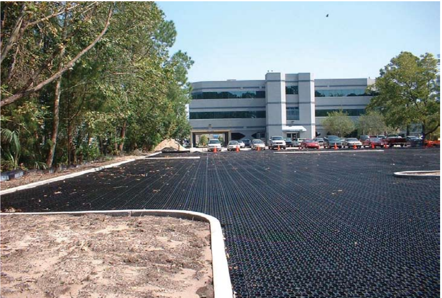
Atlantis System Installed
